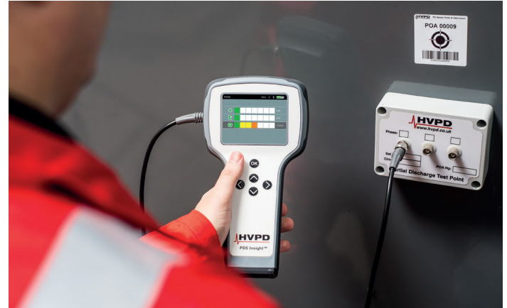
PDS Insight™ detecting PD from Phase L1 of an HFCT sensor installation
